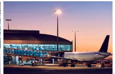
High Mast Lighting
